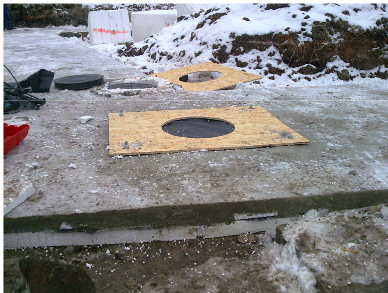
Fig. 6. The buildings vibration and seismic protection system arrangement at the pile grid level (Fig. 2).
