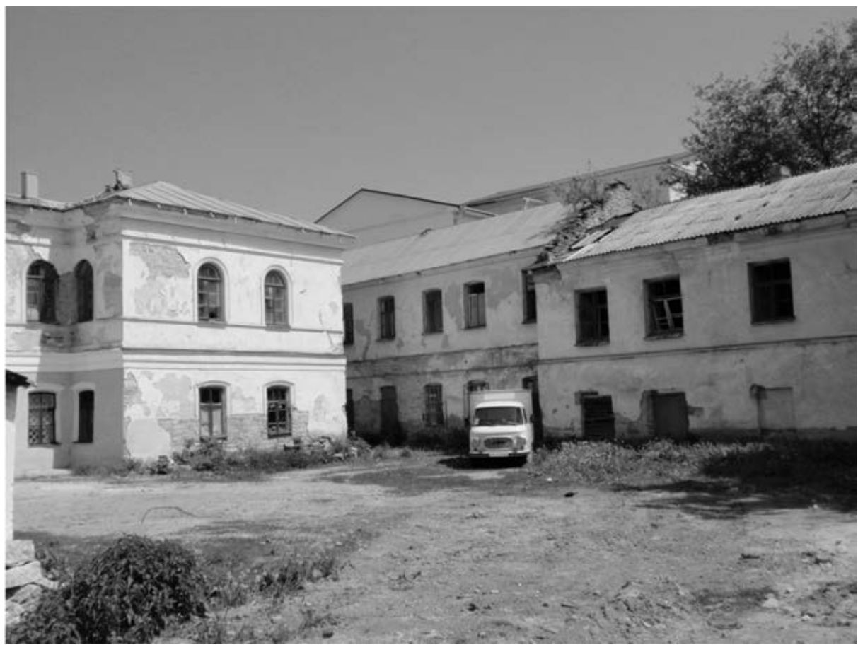
. 1. . 4. Fig. 1. General view at the house at Virmenskyi rynok square, 4.
