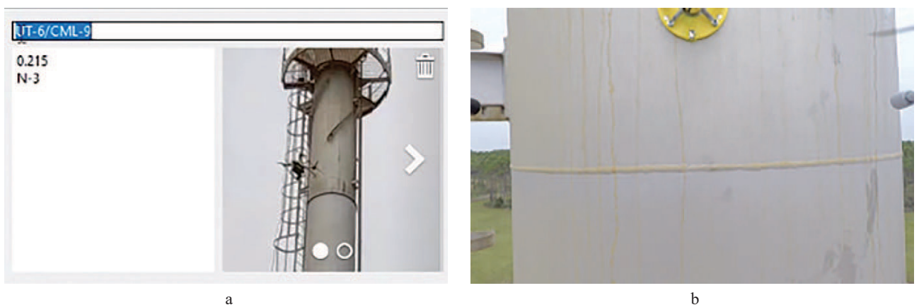
Figure 6. An example of flight details: (a) a sample UT thickness measurement reading (UT-6) at condition monitoring location 9 (CML-9) showing the lowest measurement reading out of three readings (N-3); (b) photo of the aerial robotic system making contact with the flare stack from the post-flight report (note all numbers and values are illustrative).
