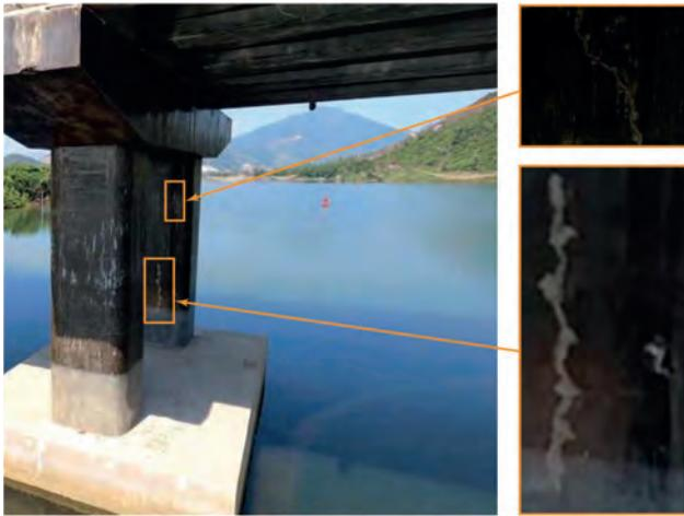
Figure 6. A snapshot from a recorded video taken by the robot. Two zoomed-in areas on the right side show the crack location
