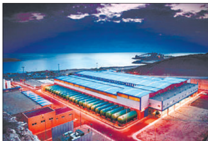
Fig. 12. Filters for seawater [82]
