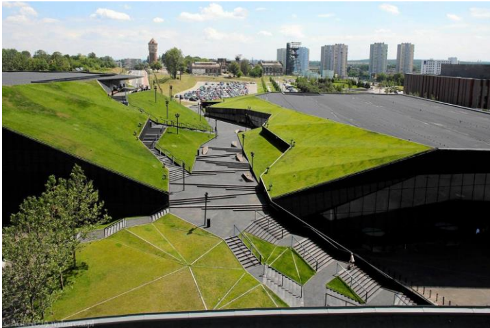
Fig. 6. Green roof over the International Congress Centre in Katowice [20]
