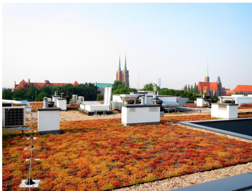
Fig. 4. Green roof at Botanica Residence in Wroclaw [18]
