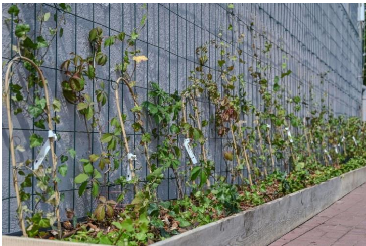
Fig. 10. Green facade created on the external wall of the City Hall building in Czestochowa [24]
