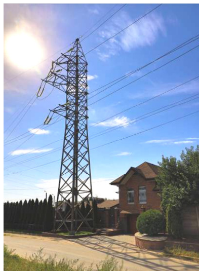
Fig. 1. Location of residential old buildings near power lines
