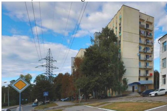
Fig. 1. A multi-storeys residential building located near a double-circuit power line
