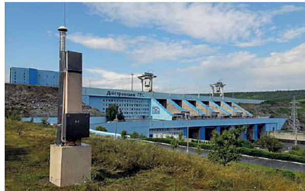
Fig. 2. General view of the Dnister HPP-1
