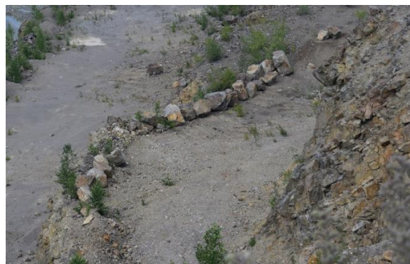
Fig. 6. Safety shaft on the quarry road (southern part of the Hnivanskyi quarry).
