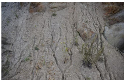
Fig. 15. Prefabricated furrows on the slopes of overburden dumps (Hnivanskyi quarry).
