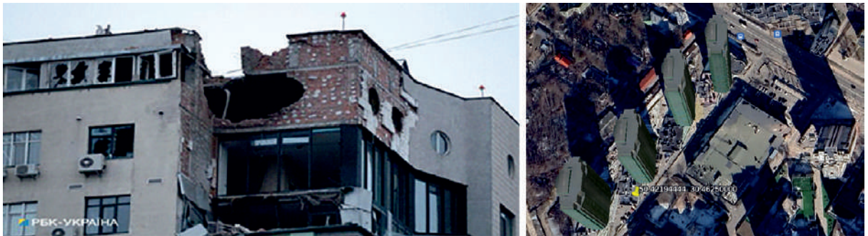
Fig. 1. A 26-story building in the Solomyanskyi district of Kyiv, damaged by debris from a downed Russian drone on the night of December 21—22, 2023. On the left is a damaged part of the house.
