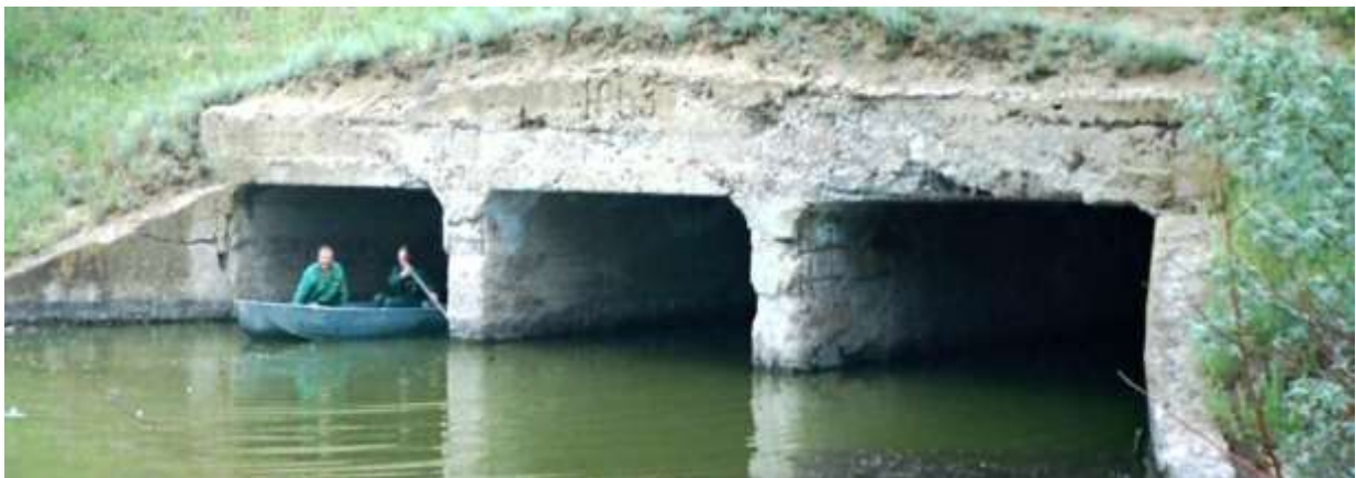
Figure 9 - Appearance of culvert
