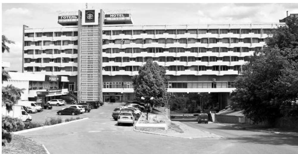
Figure 5 - An example of successful construction of a ravine on I. Akinfiieva street
