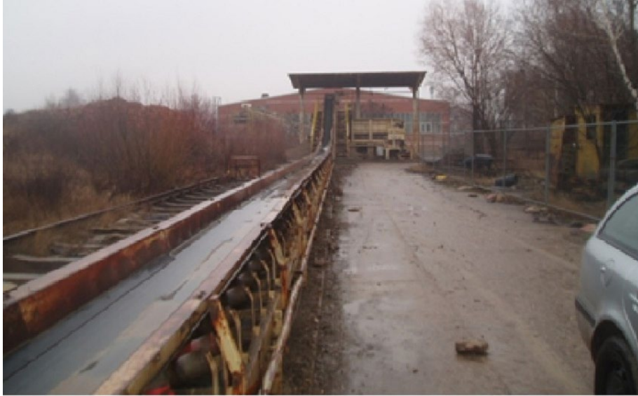
Figure 6 – Conveyor belt, Source: Ing. Jan Fiala 2019
