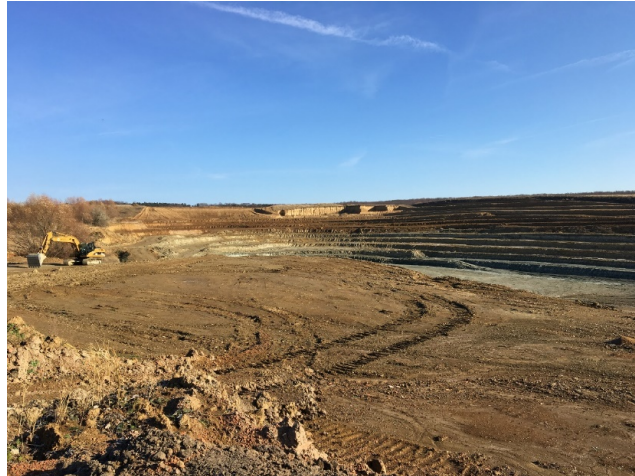
Figure 2 – Excavation premise of surface mining, Source: Wienerberger
