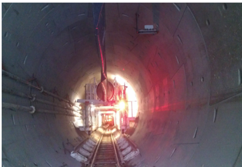
Figure 4 – Finished high-quality tunnel lining (Tashkent-2018)
