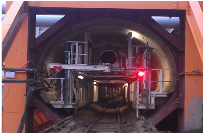
Figure 3 – The tail of the technological shield trolley (Tashkent-2018)
