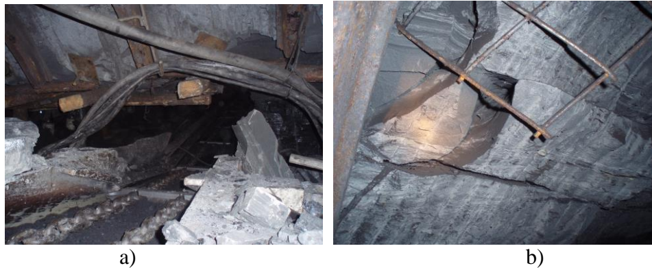
Figure 4 – Identification of rock destruction in the longwall roof (a) and in the roof of preparatory roadway (b) with the help of mine control methods (roadway 535, "Samarska" Mine)
