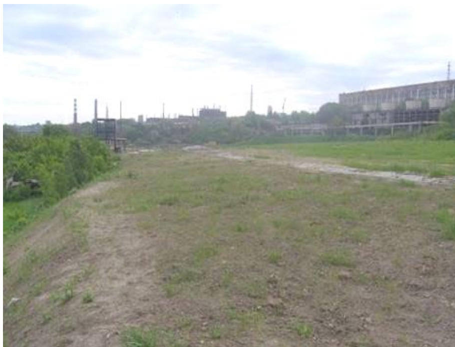
Figure 2 – Zapadnoye tailing impoundment after erosion-preventive activities
