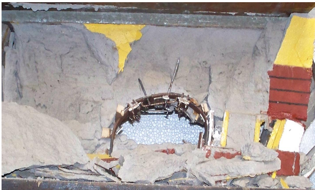
Figure 7 – Asymmetric deformation of the frame under loading for model #11
