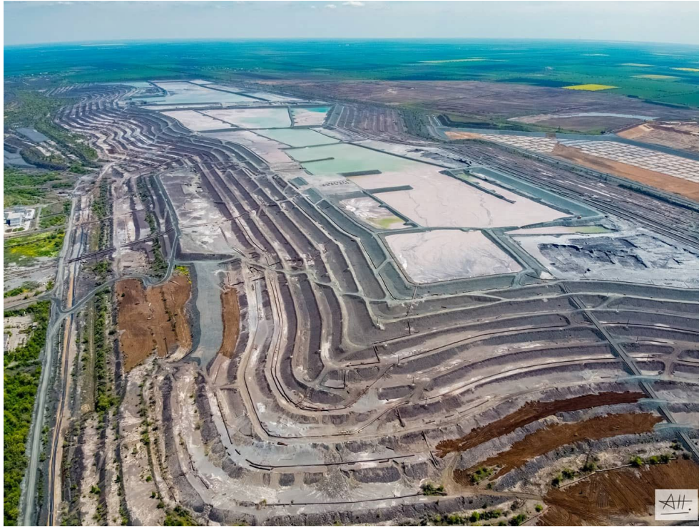
Figure 4 – Photo of the Ob'yednane tailings storage facility (A. Novak, 2021)
