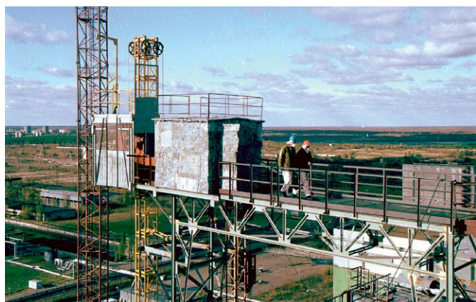
Fig. 1. Design and practical use of the shielded cabin
