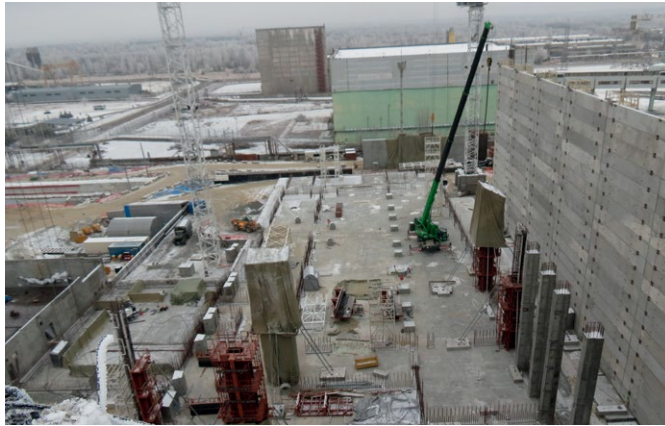
Fig. 2. Protective wall at the Shelter object site
