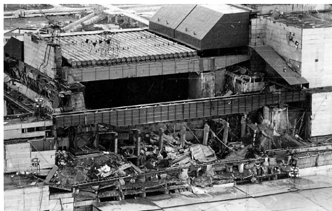
Fig. 10. Debris at the place of the Mammoth beam temporary support installation
