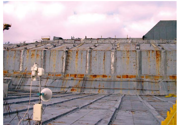
Fig. 20. State of the shields-sealers after the Shelter Object rooftop sealing completion
