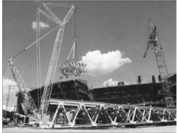
**Figure 10.** Handling of the roof girders in Donetsk
