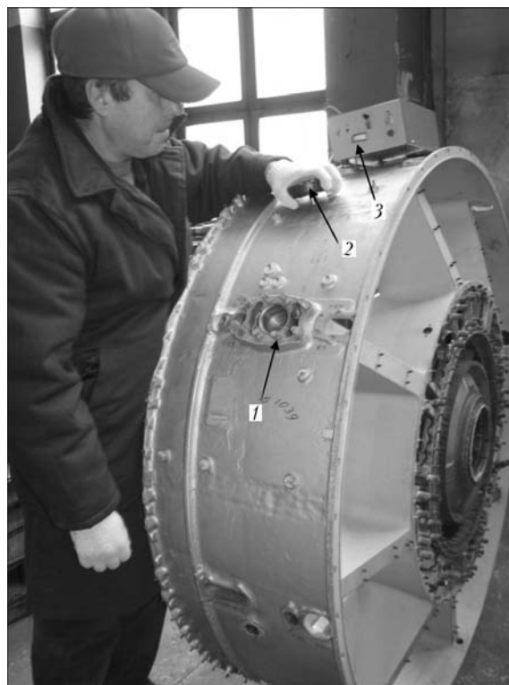
Figure 4. AEIC EDT in the zone of repair cladding of reinforcement for the flange of fastening the post cooling pipeline: 1 – reinforcement for flange; 2 – manual tool for EDT; 3 – power source for EDT
