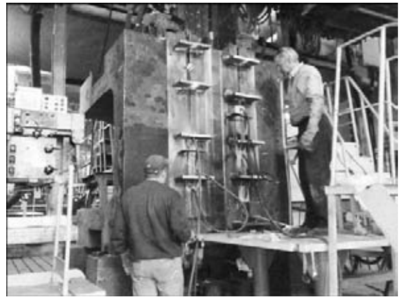
Figure 6. Moment of welding-in of the implantate at plant complex
