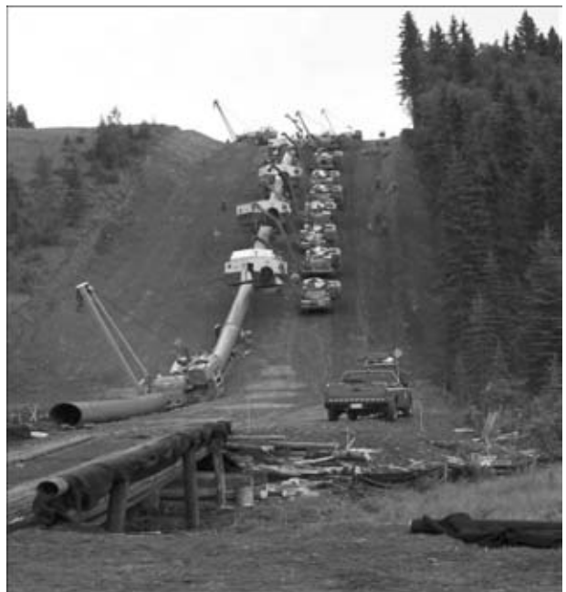
Figure 4. CRC column on the route
