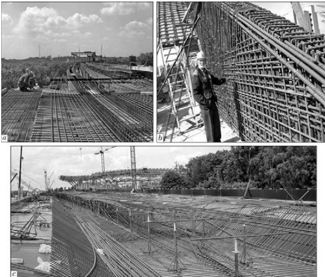
Figure 4. Structures of reinforcement cases of Podolsky bridge crossing over Dnieper River (a), bearers of VIP-sector of NSC «Olimpijsky» (b) and trestlework of terminal D of Borispol airport (c) (Kiev)
