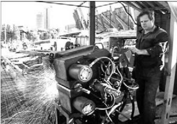
Figure 6. Suspension RBW machine K813 adjusted for reinforcement joining in construction site
