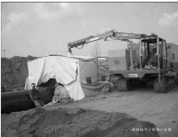
Figure 1. Building site in pipeline construction
