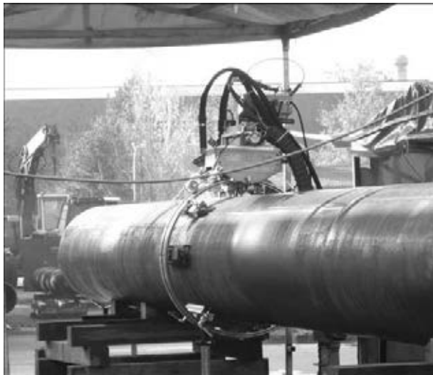
Figure 3. Entire test built-up on the pipe
