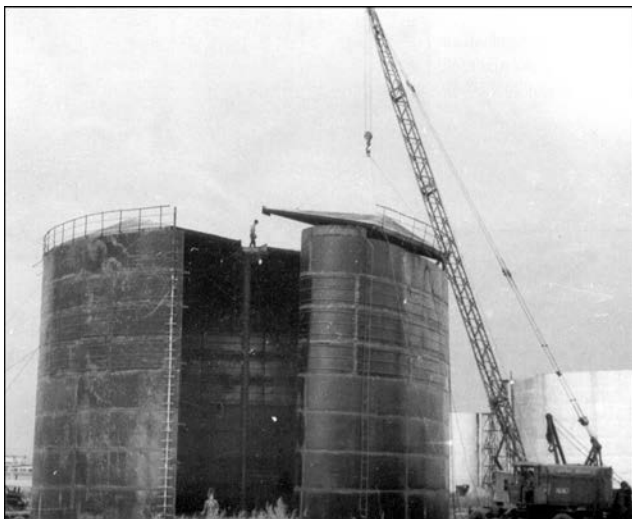
Erection of large-size tank (1948)
