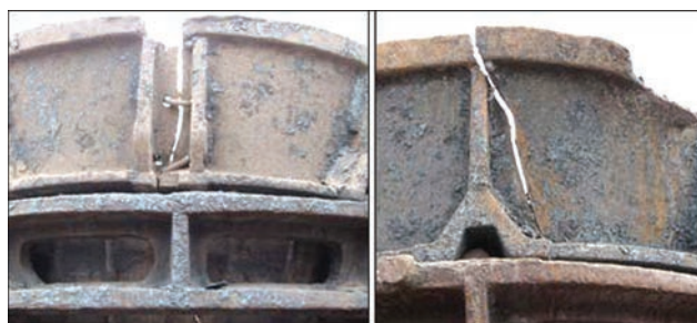
Figure 2. Cracks in slag bowls in the area of cast stiffeners
