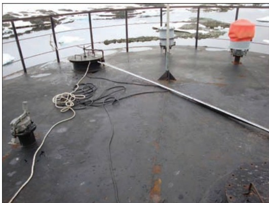
Figure 4. General view of roof of the tank RVS-200
