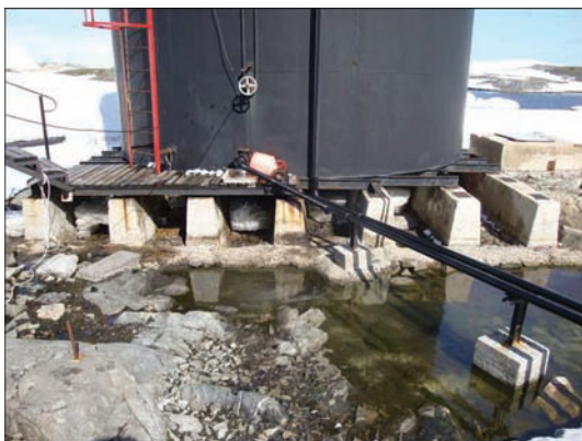
Figure 2. General view of basement arrangement of the tank RVS-200
