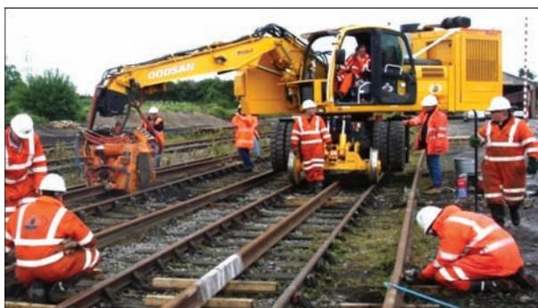
Figure 22. Mobile rail welding complex (UK)
