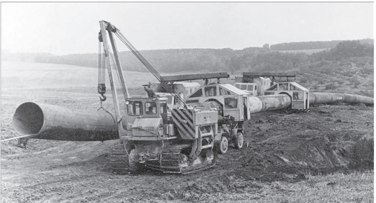
Laying the main pipeline
