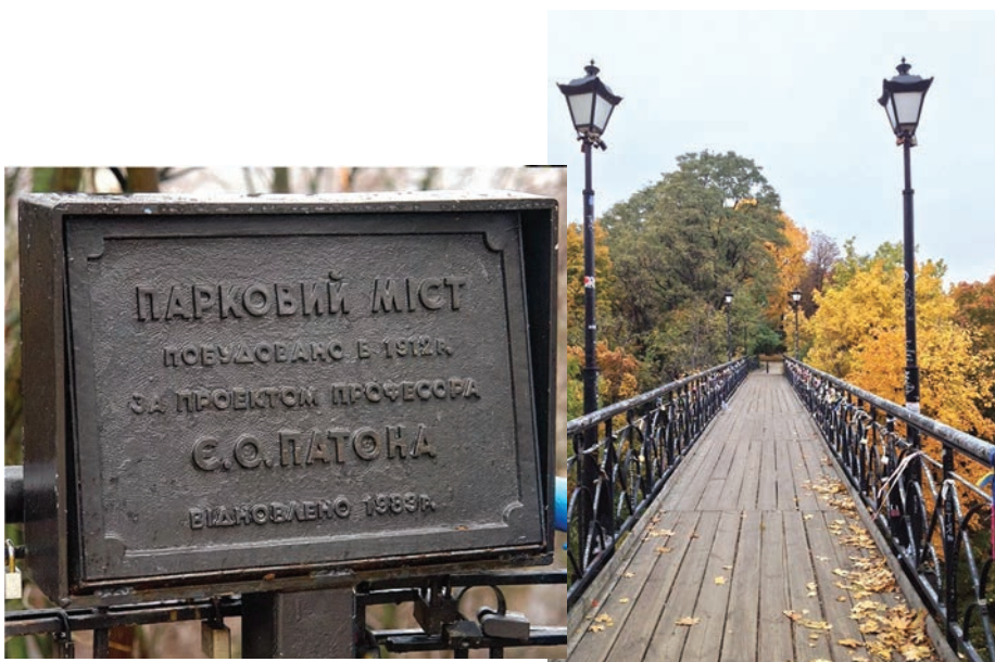
Arched bridge over Petrovskaya Alley in Kyiv, built in 1912 by E.O. Paton's design
