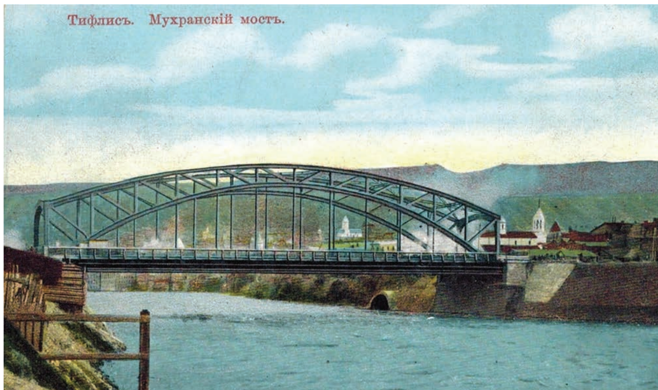
Mukhrani Bridge across the Kura river in Tiflis, built in 1908 by E.O. Paton's design
