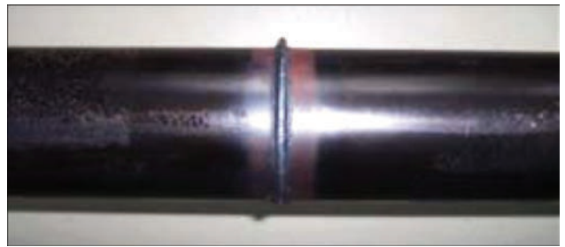
Figure 4. Uniform formation of the welded joint
