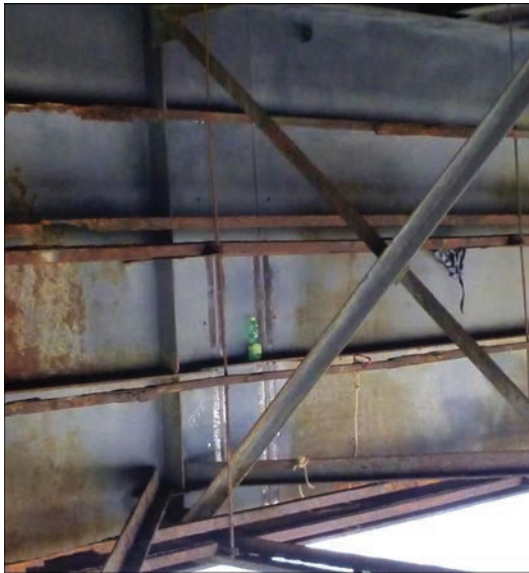
Figure 5. Example of testing butt vertical welds of the joining insert
