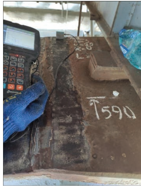
Figure 6. Example of testing butt weld in the upper girth of the joining insert
