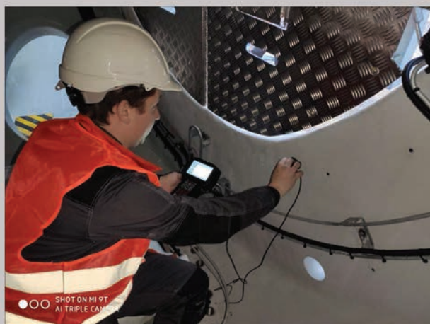
Ultrasonic testing of wind turbine hub
