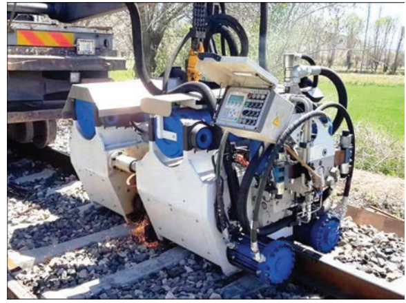
Figure 6. Welding head AMS100
