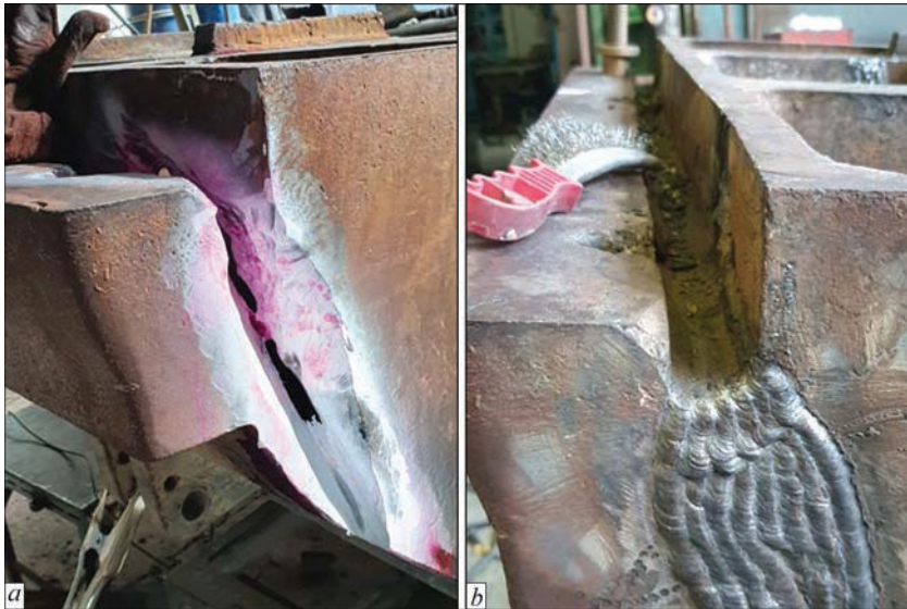
Figure 5. General view of repair of crack No. 2 on the front wall after mechanical edge preparation (a) and after welding (b)
