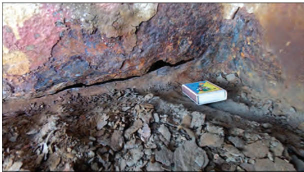
Figure 2. Crack formed in the zone of corrosion thinning of the weld in the span F46 of the main beam No. 4
