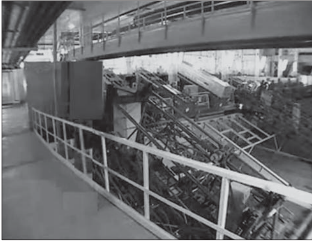
Fig. 2. Module testing stand of transmission modules manufacturer
