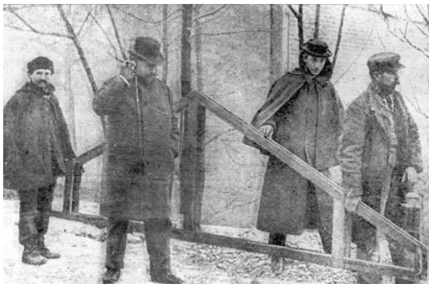
Photo 1. One of the first locators to search underground communications, 1910.
