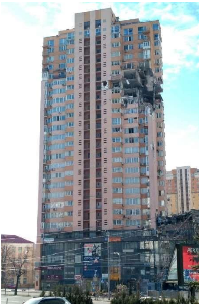
Fig. 6. General view of the building at 6A Lobanovsky Avenue after the rocket impact on April 26, 2022
