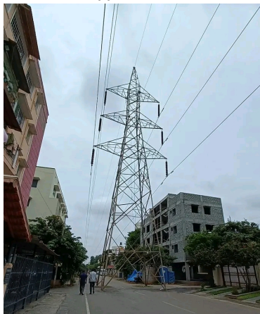
Fig. 1. Residential buildings located close to power line
